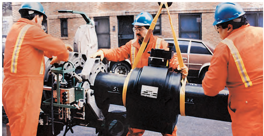
12" Poly-Gas® valve fusion operation
